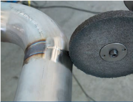
Removing welding discoloration.
