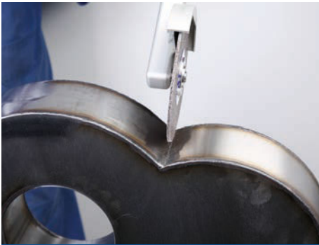
Removing TIG welds.
